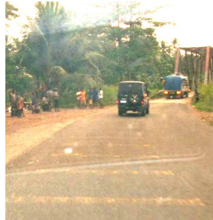
Figure 5.2 Poorly maintained yellow bar markings on the Hiritano Highway
